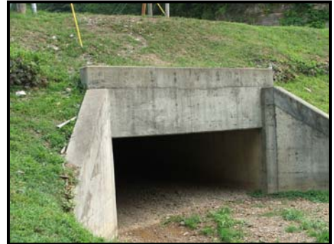
Culverts under KY 1460 (top) and KY 1426 (bottom)
